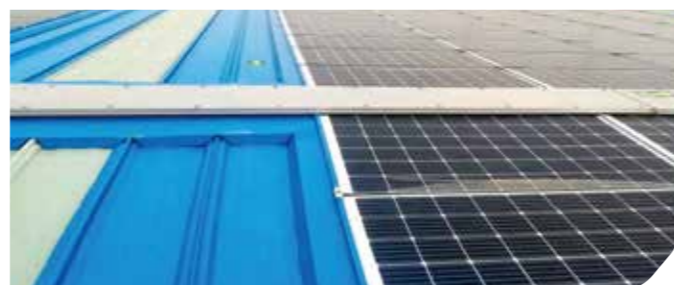
Risen Energy Jiangsu 2.1 MW
